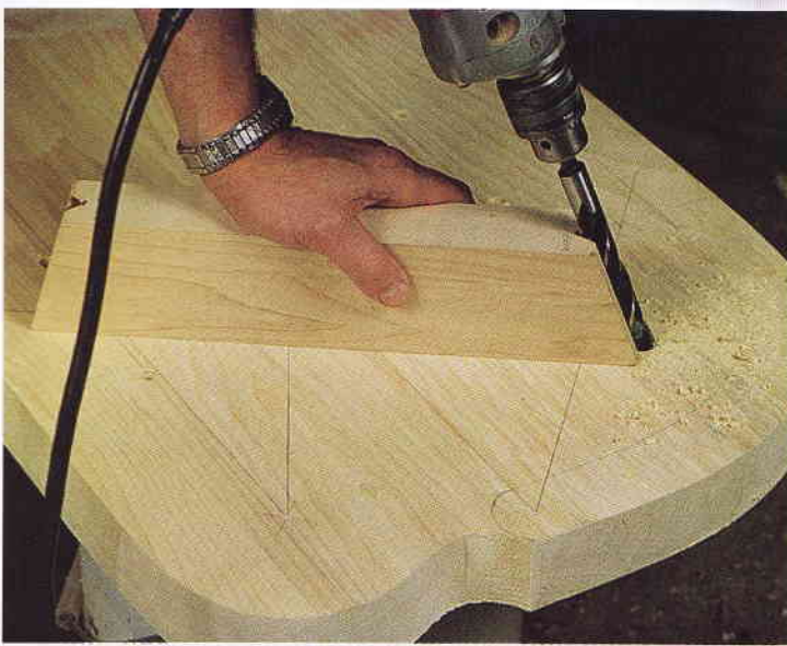
The leg and stump holes are bored from the top down, so any tearout is hidden on the bottom. The drill is guided by a notched scrap of 2x3x8 hardwood, crosscut on one end to the desired angle. Pencil lines drawn on the seat indicate the direction in which the angled legs lean.
