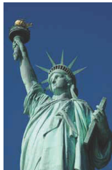
Figure 26.14 The green patina of the Statue of Liberty is due to the surface formation of copper hydroxycarbonate and hydroxosulfate compounds. A major restoration of the statue's surface ended in 1986.
