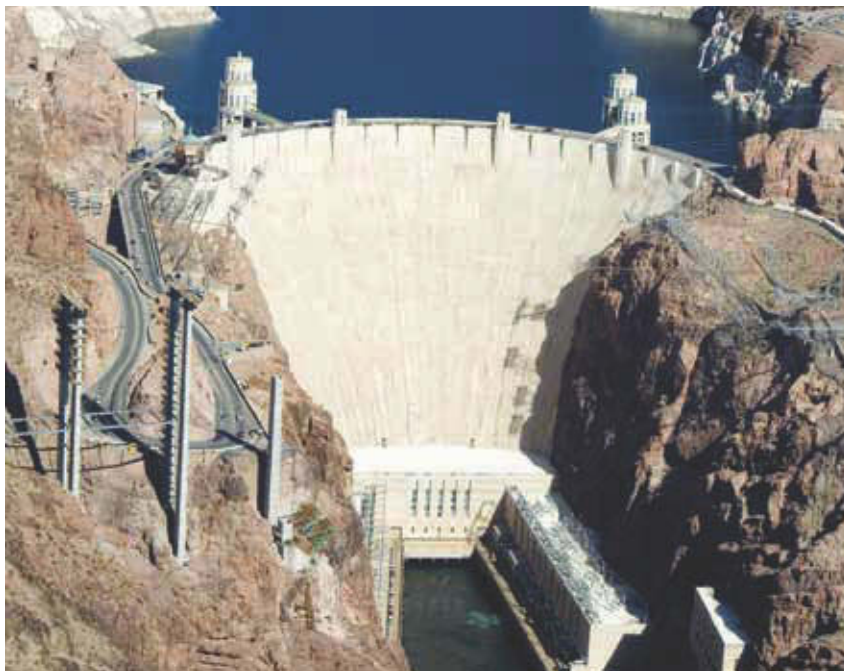
Figure I.12 Hoover Dam at Lake Mead. The potential energy of the water in Lake Mead is converted to electrical energy when it drops from near the lake surface to the bottom of the dam. The falling water drives the turbines that are within the dam and generates electricity.
