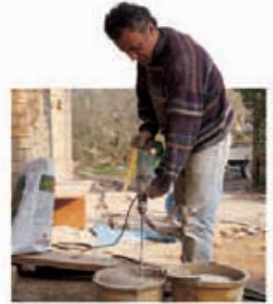
建築屋 kenchiku-ya construction worker
