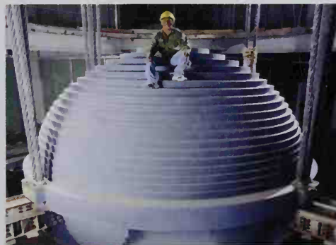
■ Construction worker on Taipei 101 mass damper.
