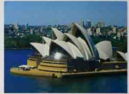
■ Concrete structures allow almost any kind of shape. Shell structures like the roofs of the opera house in Sydney are reinforced with steel rod mats and can span wide spaces without further support.
