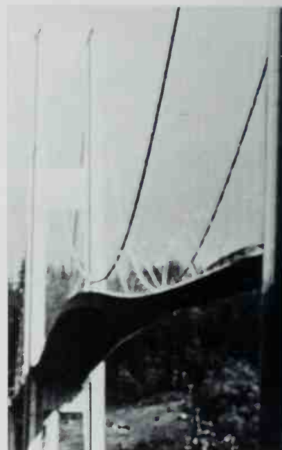
■ Tacoma bridge vibrating violently due to hurricane winds causing a violent oscillating motion.
