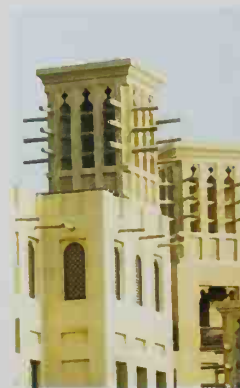
■ Taking advantage of natural thermal currents, windcatchers provide effective cooling while ensuring sufficient ventilation.
