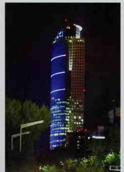
■ There are 98 seismic dampers set into the reinforced concrete and dual steel structure.
