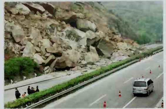
■ Following rockslides, roads can often become impassable due to undercutting or large taluses blocking the traffic.
