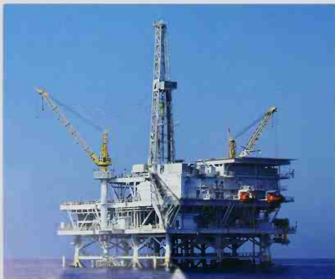
■ Rigs extract oil and natural gas through holes drilled in the ocean bed. These structures may be attached to the ocean floor, consist of an artificial island, or be a floating platform.
