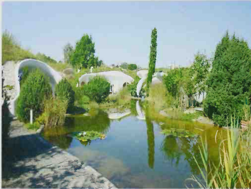
■ The grass-covered roof of this "eco-villa" in Switzerland provides excellent insulation, while the pond serves as a natural habitat for local flora and fauna.
