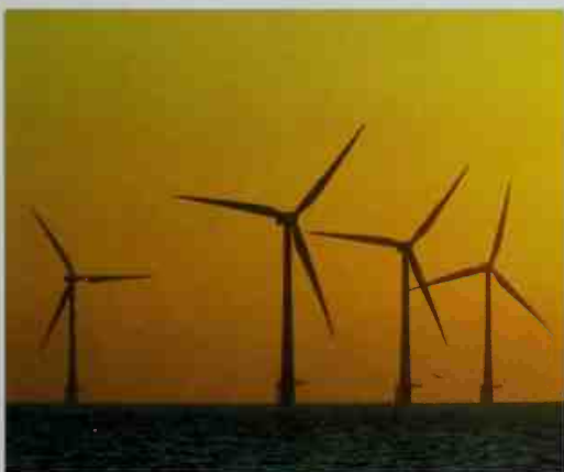
■ Germany's Borkum West II is set to be one of the world's largest offshore wind parks when it is completed in 2009.
