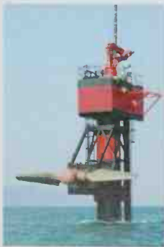
■ Seafloor turbines (here raised out of the water for maintenance) have 33-foot-tall mill-turbine blades
