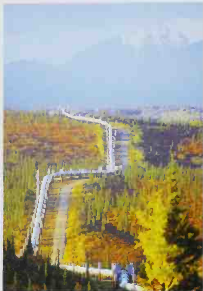
■ Oil and natural gas pipelines in extreme climates must be well protected against corrosion.
