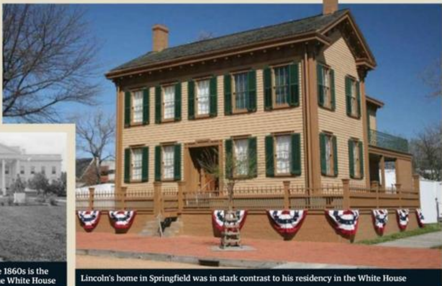
Lincoln's home in Springfield was in stark contrast to his residency in the White House
